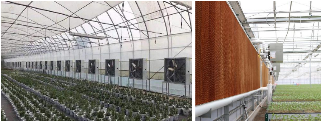
Gambar 6. Sistem pendinginan fan and pad cooling system dan evaporative cooler (Sumber: https://id.exhaustfanchina.com/memproyeksikan/kipas-ventilasi-rumah-kaca/ dan https://www.growerssupply.com/prod/108997.html )
