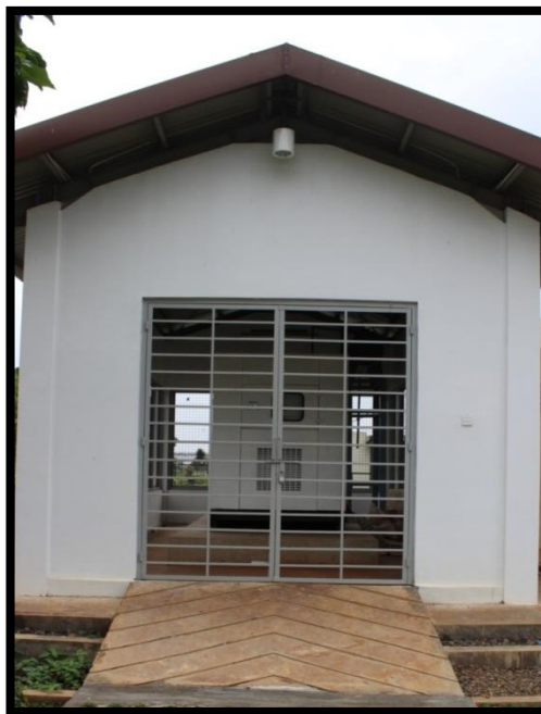
Gambar 5. Fasilitas Generator/Power Supply
