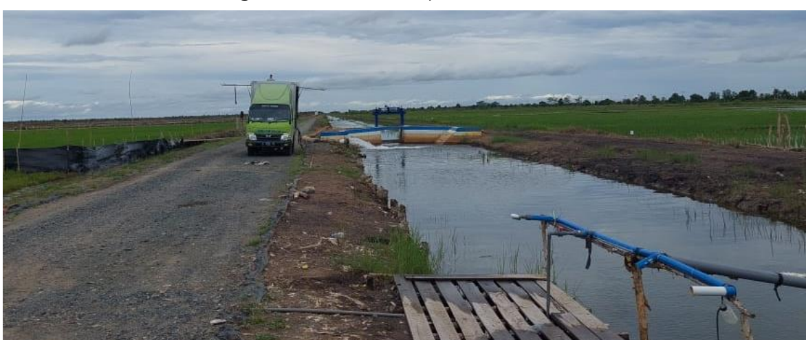
Gambar 4. Irigasi di lokasi food estate Kec. Dadahup, Kalteng
