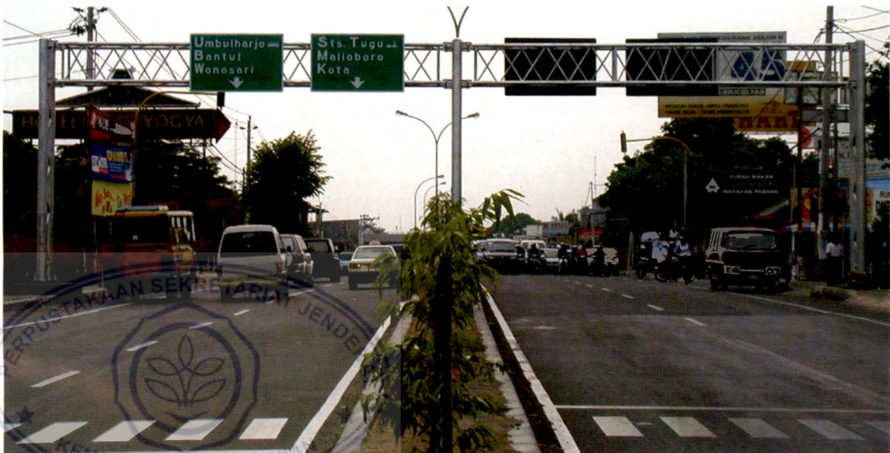
Land transportation facility.
