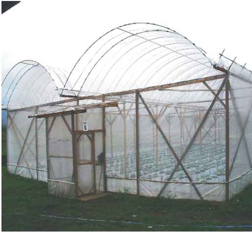
Gambar 2. Rumah plastik kayu-metal ( Wood-metal type plastic house )
