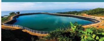
Embung/Long Storage/ Dam Parit
