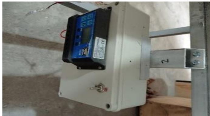
Gambar 25.Pemasangan Solar Controller
