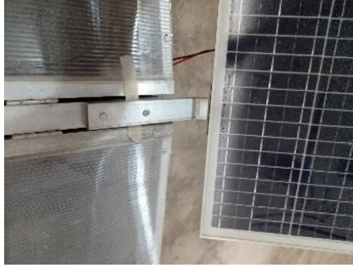
Gambar 24.Pemasangan Panel Surya
