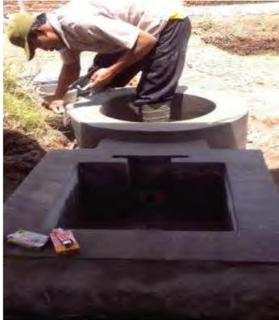
**Gambar 2. Inlet biogas**
